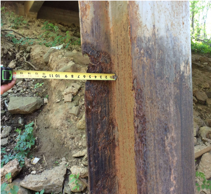
PHOTO 1 Description Bent # 2 right steel pile column with up to 2 1/2" section loss to the flange.
