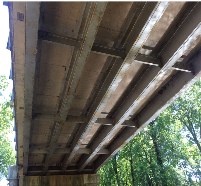
PHOTO 1 Description Failing paint system.
