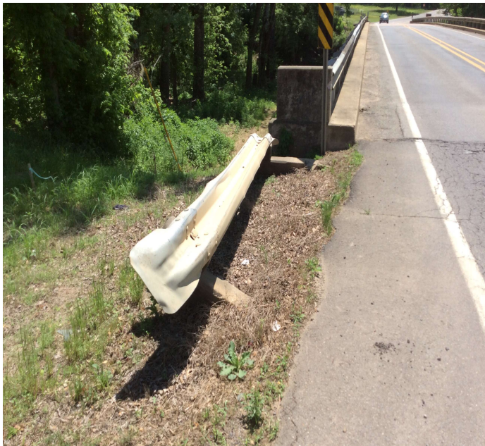
PHOTO 1 Description Northeast approach guardrail damage.
