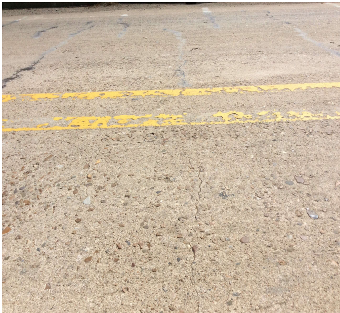
PHOTO 1 Description The driving surface of Span 3 has sealable cracking.
