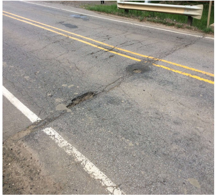
PHOTO 2 Description The approach roadway at Bent 9 (North abutment) is cracked and has potholes at the bridge end.
