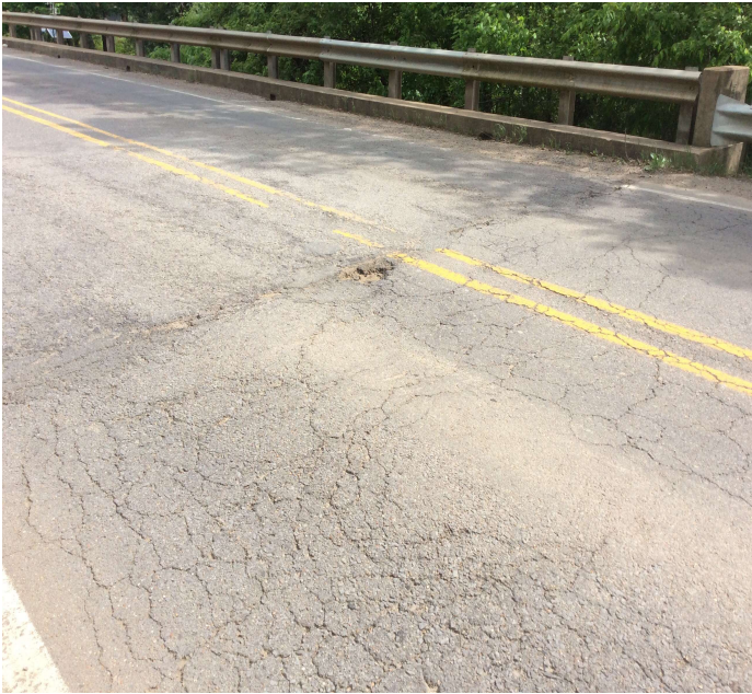
PHOTO 1 Description The approach roadway at Bent 1 is cracked and has potholes at the bridge end.
