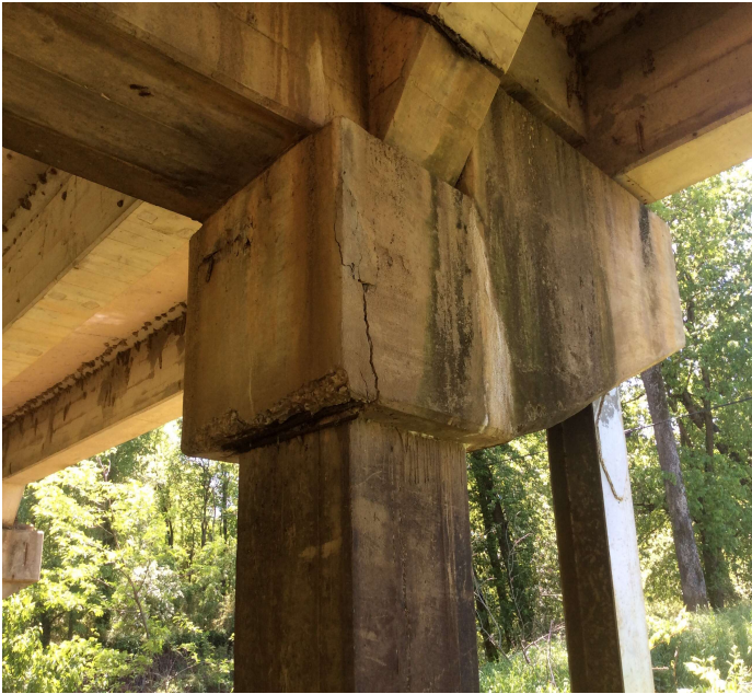
PHOTO 1 Description Bent # 5 left cap cracking and spalling with exposed reinforcing steel.
