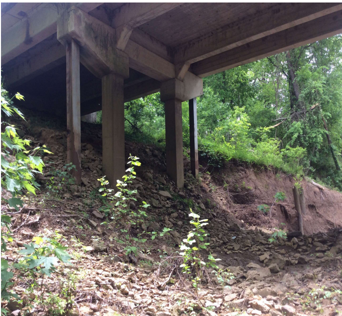
PHOTO 1 Description Embankment erosion at Bent 2 that has removed approximately 3' of embankment material from the base of the Columns .
