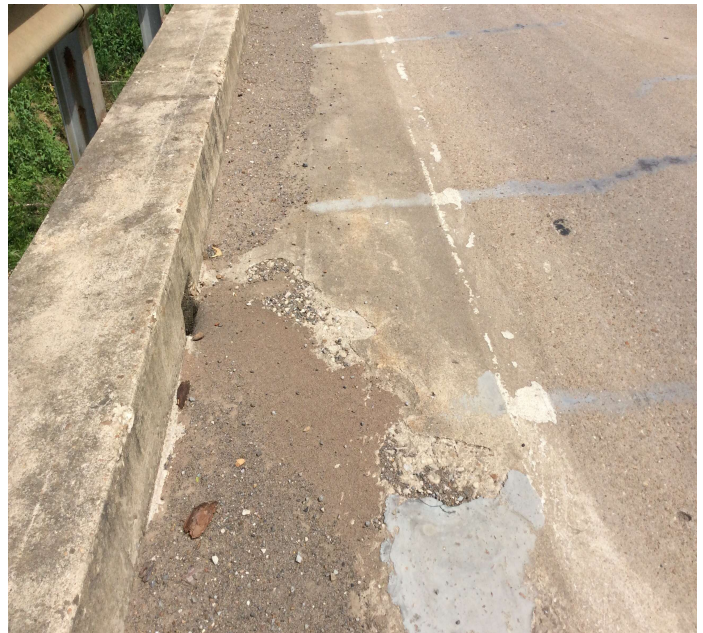
PHOTO 2 Description Span 3 has sealable transverse deck cracking and light scale in the gutters.
